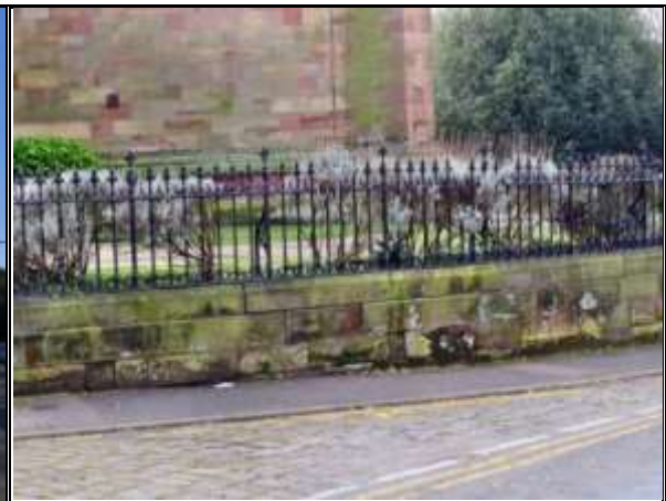
Photograph 8: Listed Railing and Wall, St Mary's Church
