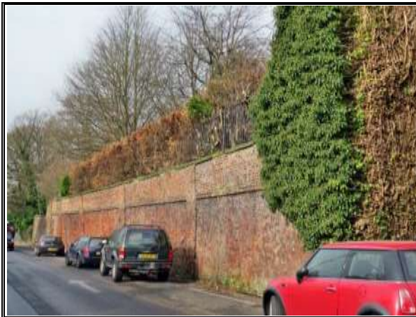
Photograph 107: Retaining Wall of Kirklee from Church Brow
