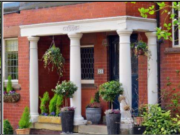
Photograph 84: Entrance Porch to The Red House, 51 Langham Road
