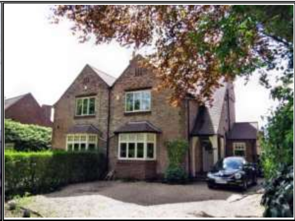
Photograph 80: Weynefleet, Grange Road
