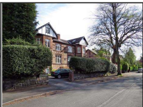
Photograph 130: Boundary treatment on Winton Road
