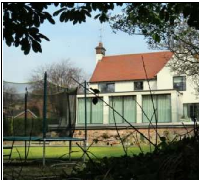
Photograph 149: Modern Extension to Rear, Talbot Road:
