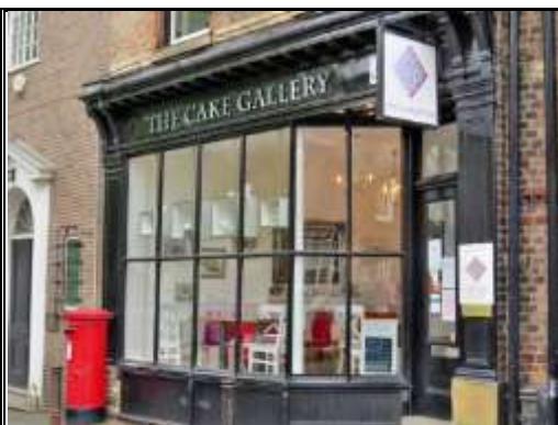
Photograph 18: Retention of Historic Shop Fronts, The Polygon
