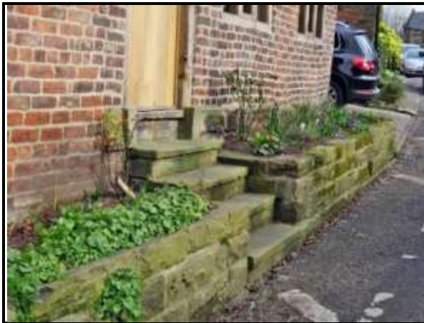
Photograph 45: Flower Beds & Lack of Pavement on Church Brow
