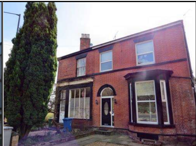
Photograph 140: Inappropriate Door and Windows, 33 Langham Road
