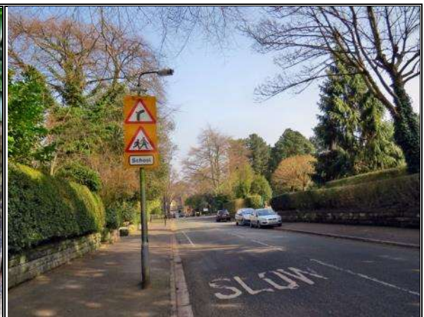
Photograph 110: Traffic Signs and Road Markings on The Firs
