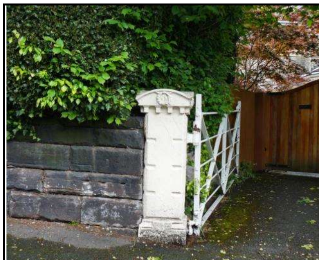
Photograph 165: Original Gatepost with Intrusive Gate Beyond, Larkhill, Heald Road
