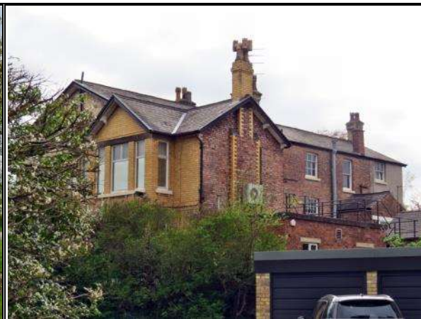
Photograph 104: Rear Elevation of Byefield and Lynwood
