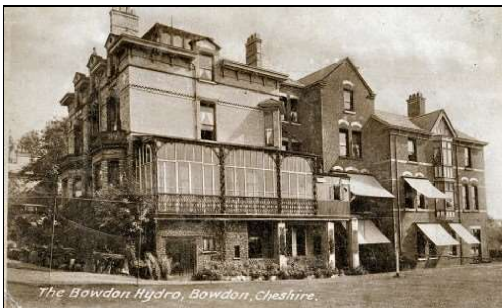
Photograph 3: Bowdon Hydro, 19 th Century. (Trafford Lifetimes, TL1561)
