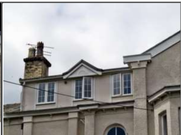
Photograph 98: Roof Extension, 7 The Firs
