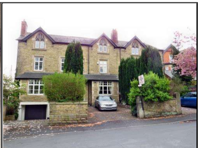
Photograph 144: Garage in Basement, West Road
