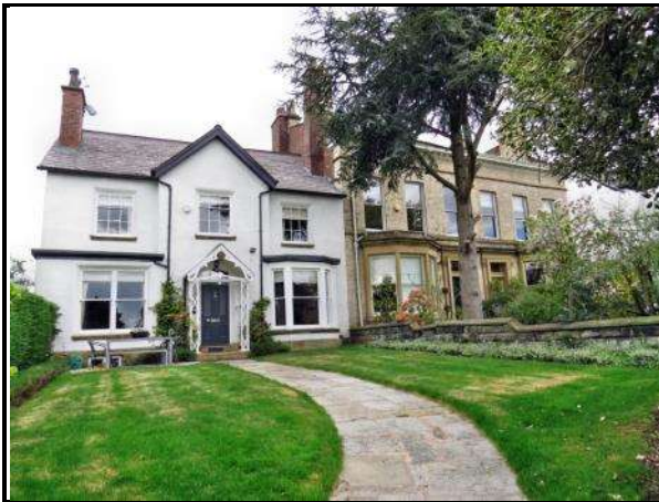
Photograph 63: Willow Cottage and 6-8 East Downs Road
