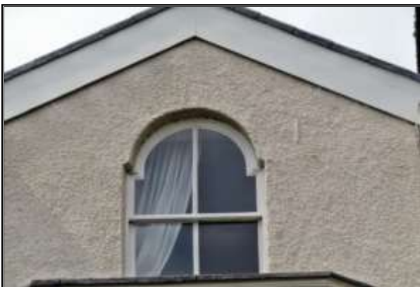
Photograph 97: Semi-Circular Arched Window, 15 The Firs
