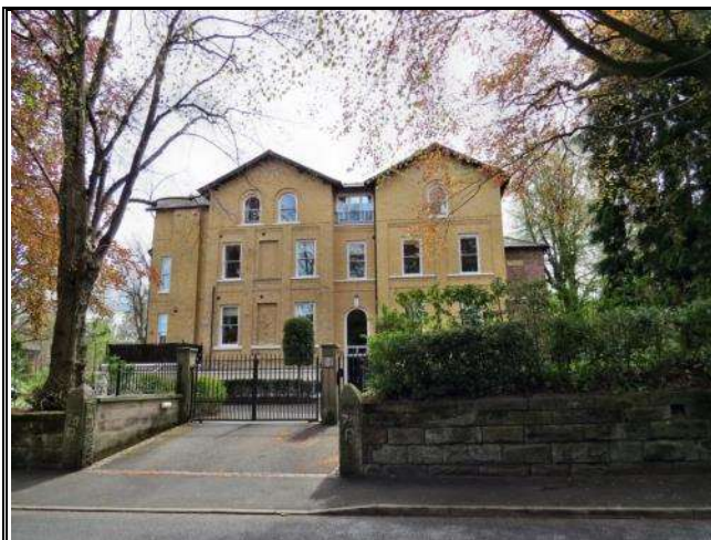
Photograph 141: Loss of Character Through Excessive Extension and Hard Landscaping (Chesham Place)
