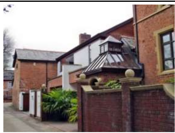
Photograph 60: New Development to Rear of 50-52 Stamford Road
