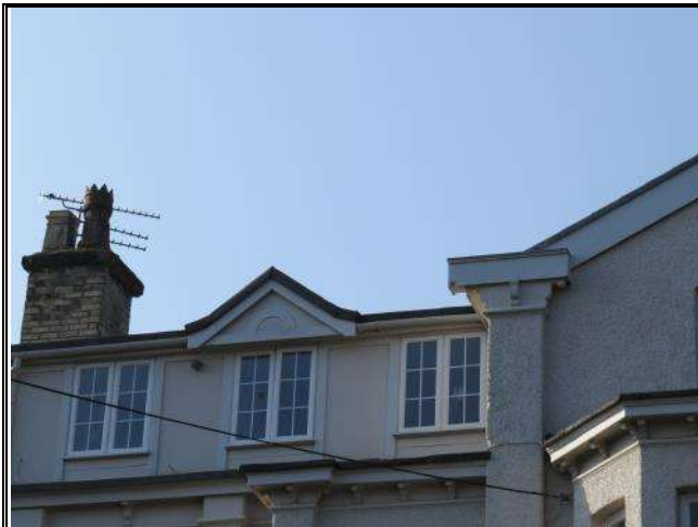
Photograph 139: Roof Extension, The Firs
