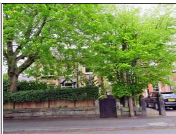
Photograph 21: Boundary Wall, Fence, Stone Gateposts (11 Stamford Road)
