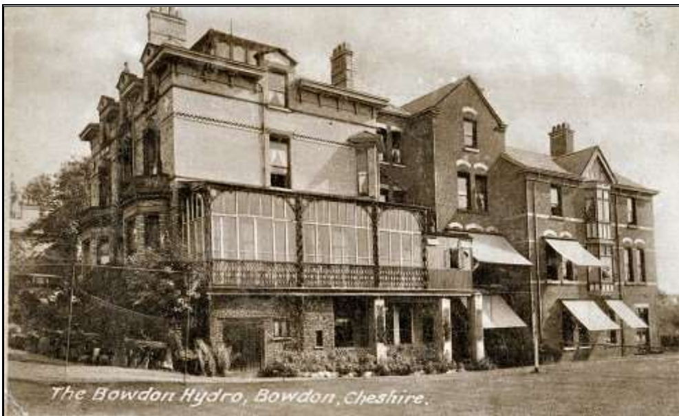
Photograph 3: Bowdon Hydro, built by 1871 (Trafford Lifetimes, TL1561)
