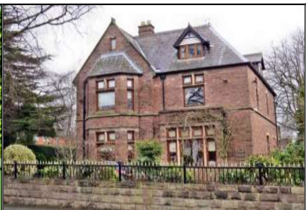
Photograph 116: The Manse, 7 Enville Road
