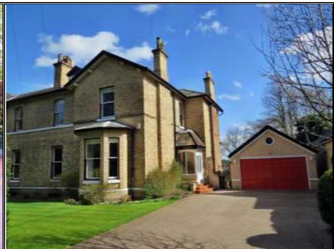
Photograph 146: Intrusive Colour of Garage Door
