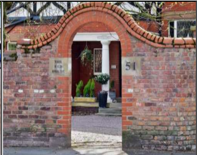
Photograph 160: Brick Wall, Red House, Langham Road
