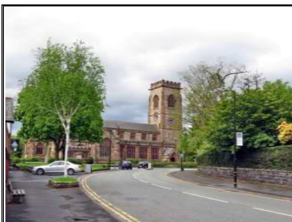
Photograph 27: View of Church from The Firs
