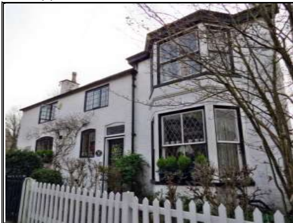
Photograph 29: The White Cottage, 10 Church Brow
