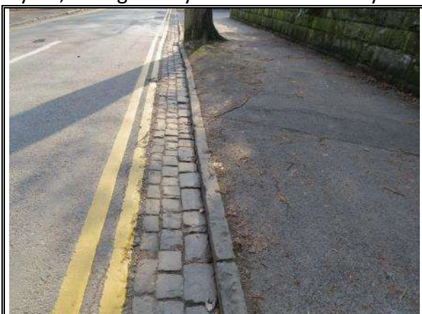
Photograph 121: Setts and Yellow Lines on Enville Road
