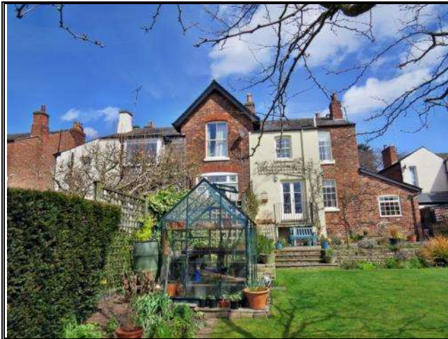
Photograph 147: Rear view with different windows and surfaces (53-65 Langham Road)
